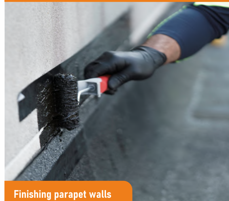
Sealing of vertical-horizontal joints
